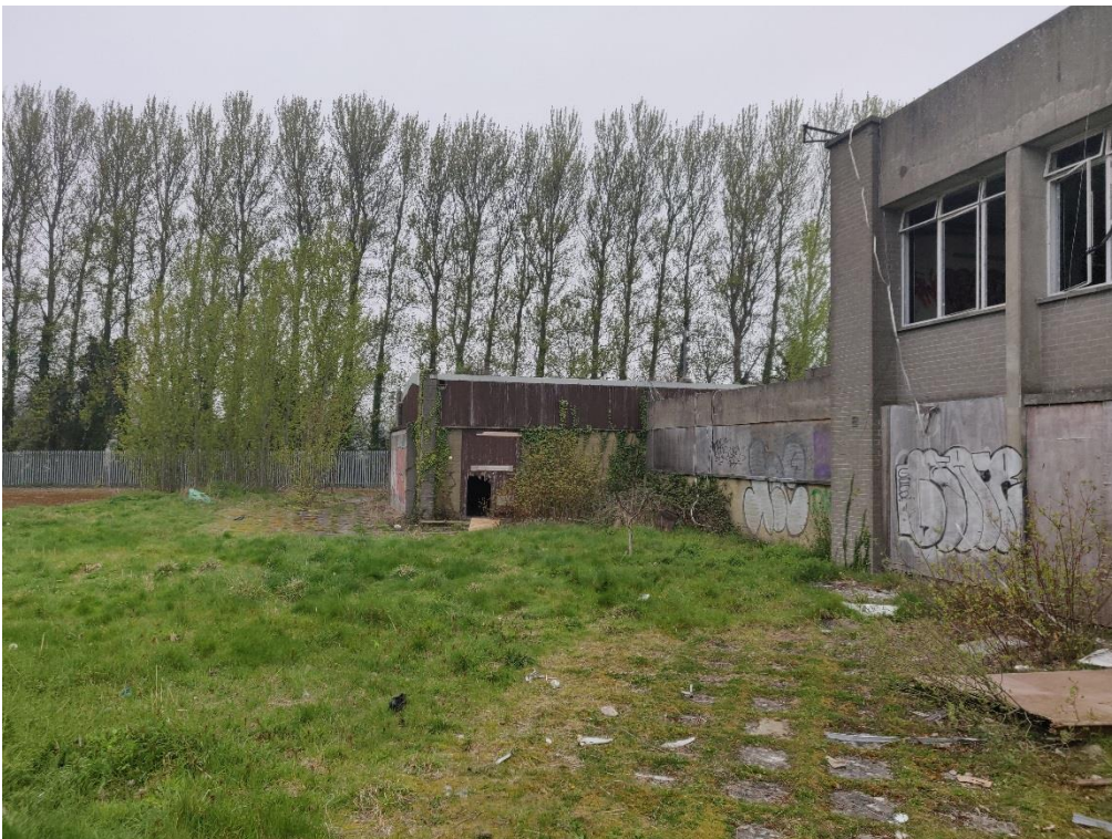
Figure 6.5 – End of Building 3 & 4: Storage Warehouse: East Elevation
