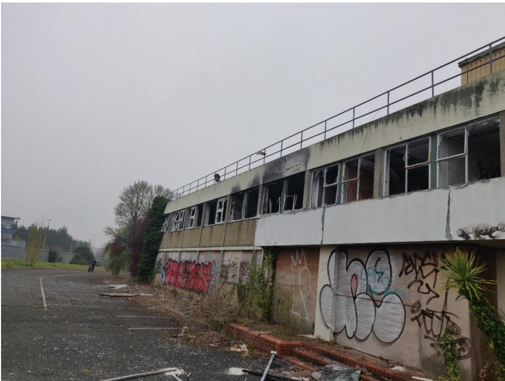
Figure 6.3 – Building 2: East Elevation
