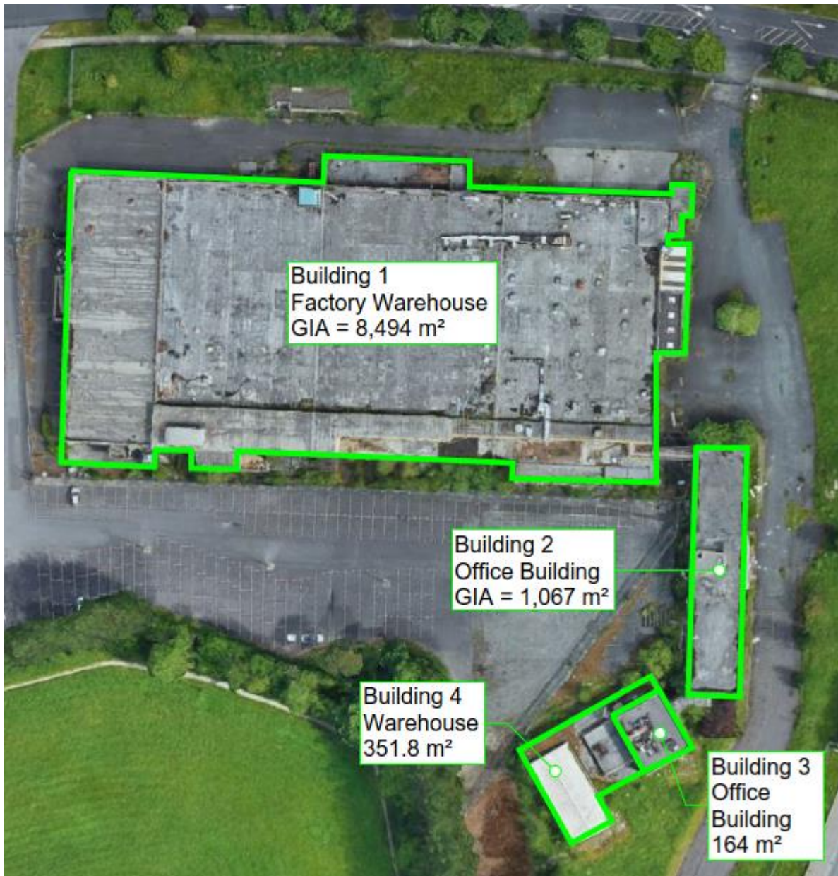
Figure 6.1 – Aerial View of Site Showing Buildings to be Demolished and Building Footprints
