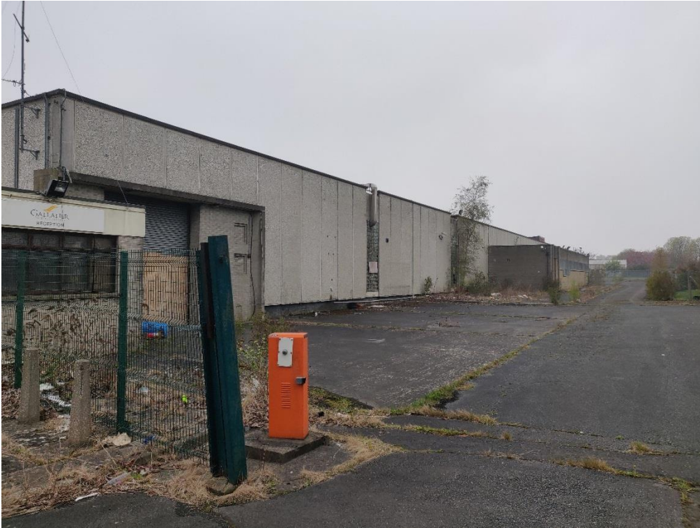
Figure 6.2 – Building 1: Factory Warehouse: North Elevation.
