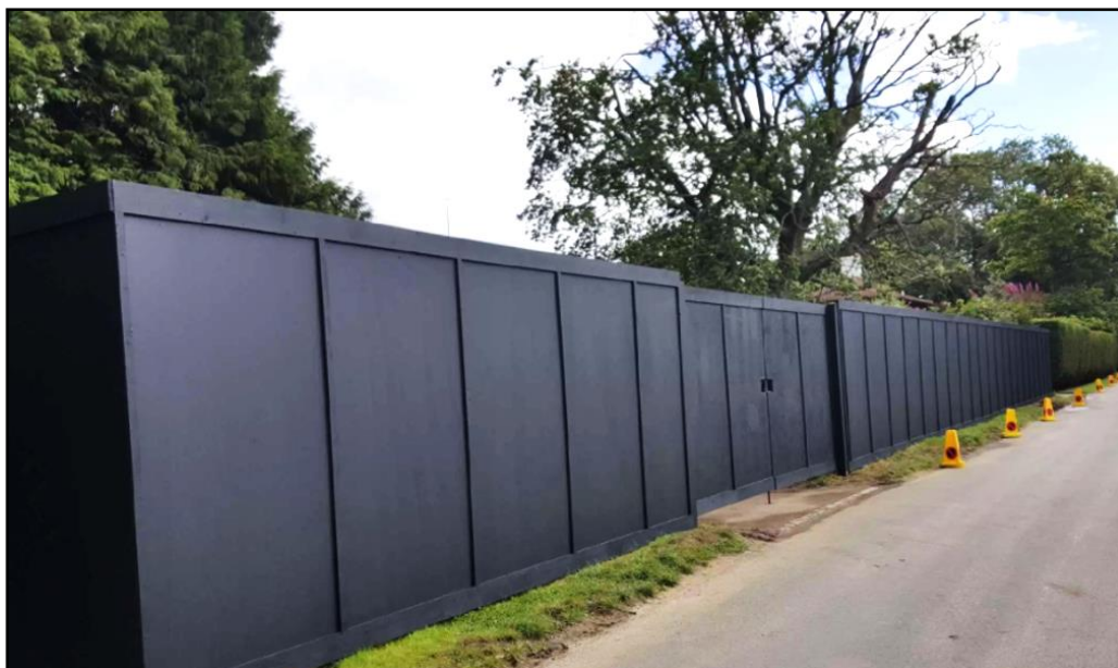
Figure 9.1 – Typical Site Hoarding Arrangement
